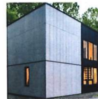
6. NATURAL FINISH FIBRE CEMENT CLADDING
